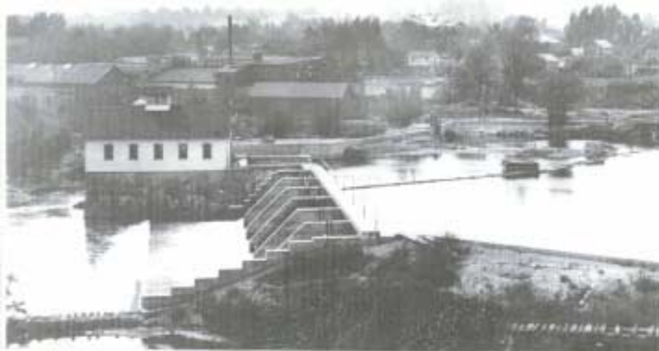
Original hydroelectric dam structure. Photo taken facing west (46).
