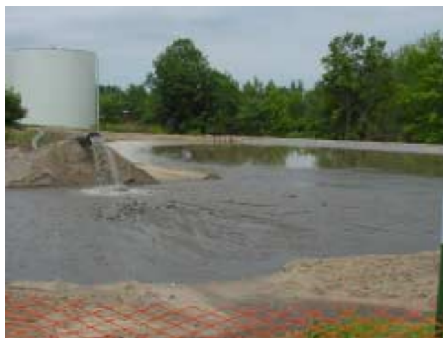
Sediment collection basin. Photo taken facing northeast, July 6, 2000 (46).
